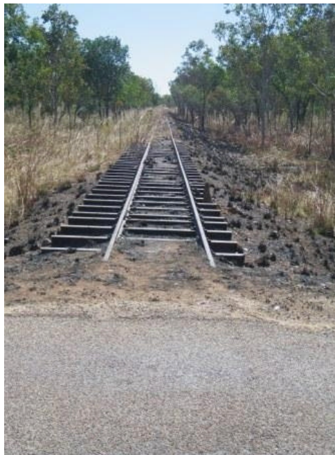
The dual punched sleepers at Katherine, Photo Adelaide River
