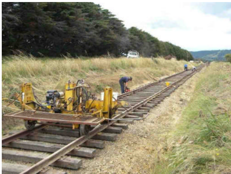
Track work towards Yarra Glen - Photo YVR
