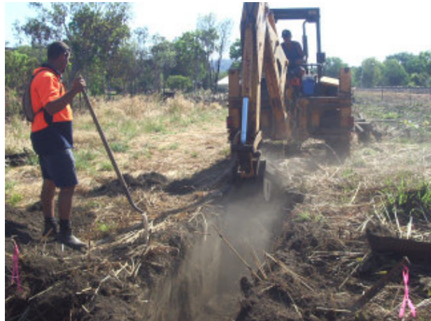
Peter Bruce clearing out the northern half of the pit
