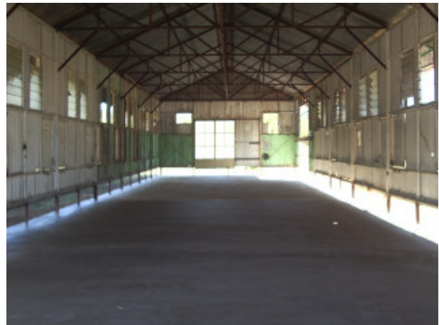
The freshly-poured concrete floor, thanks to a grant from the Coomalie Council
