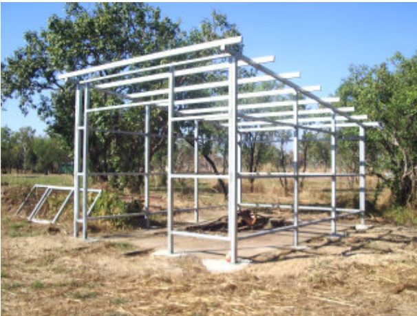
The fully erected steel frame on 24 May.
