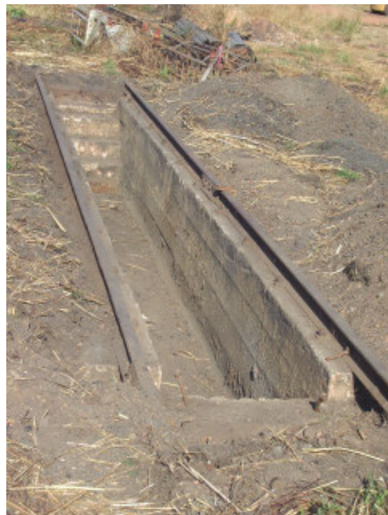
The excavated ash pit on 21 June See also 1944 photo by Jim Harvey on page 19
