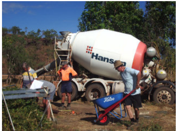
Kerry Moran barrowing the concrete to the foundation holes on 16 May 2009.
